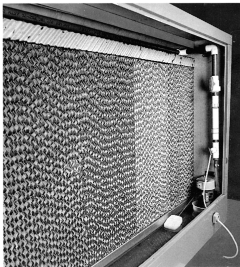
Internal View Evaporative Cooler
